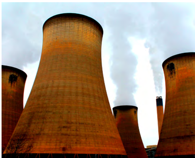
Figure 12.24 Cooling towers at the Drax power station in North Yorkshire, United Kingdom (credit: Les Haines, Flickr)
